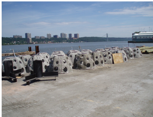
D-2: Reef balls on site prior to installation
