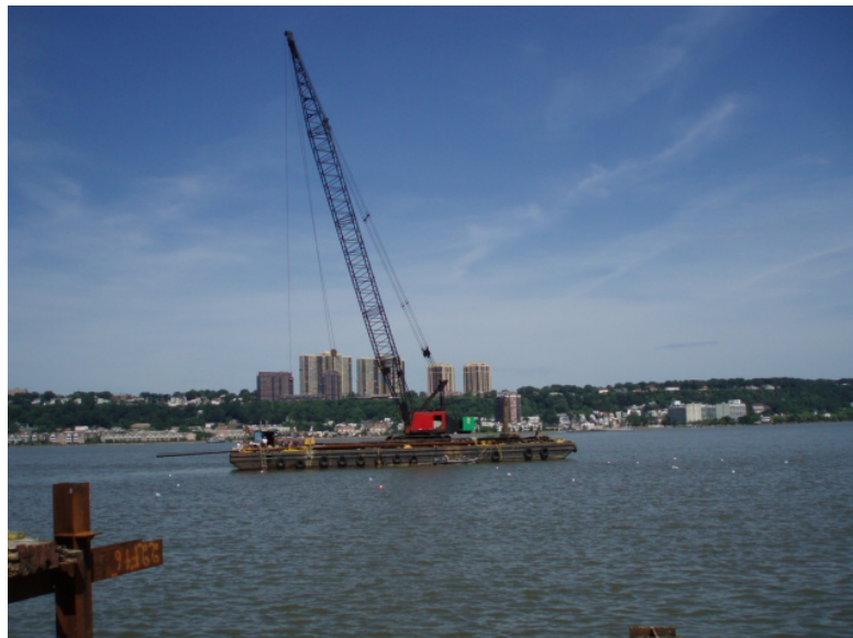
D-4: Installation of reef balls. The white buoys in the water indicate reef ball locations
